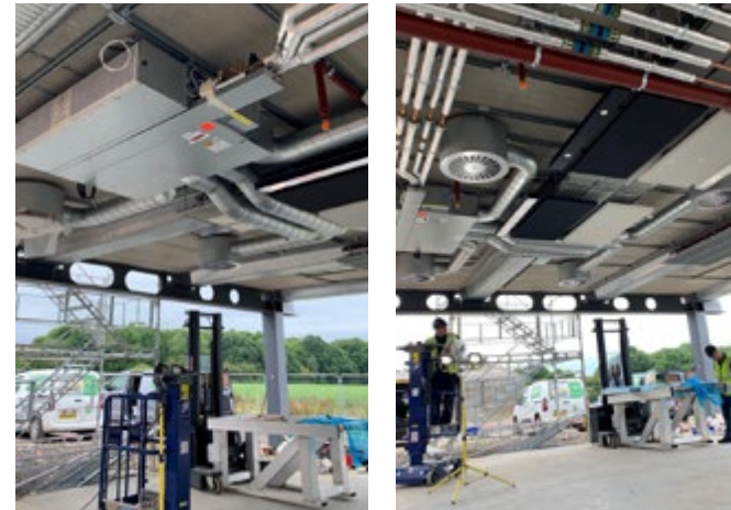
Installation of prototype M+E cassettes.
