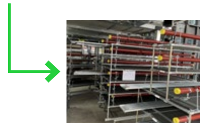
MEP cassette transport and installation
