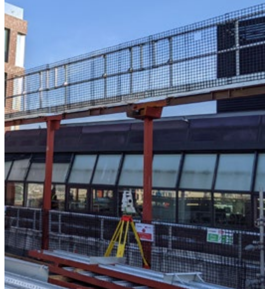
Microcolumns with temporary handrails installed at The Forge.
