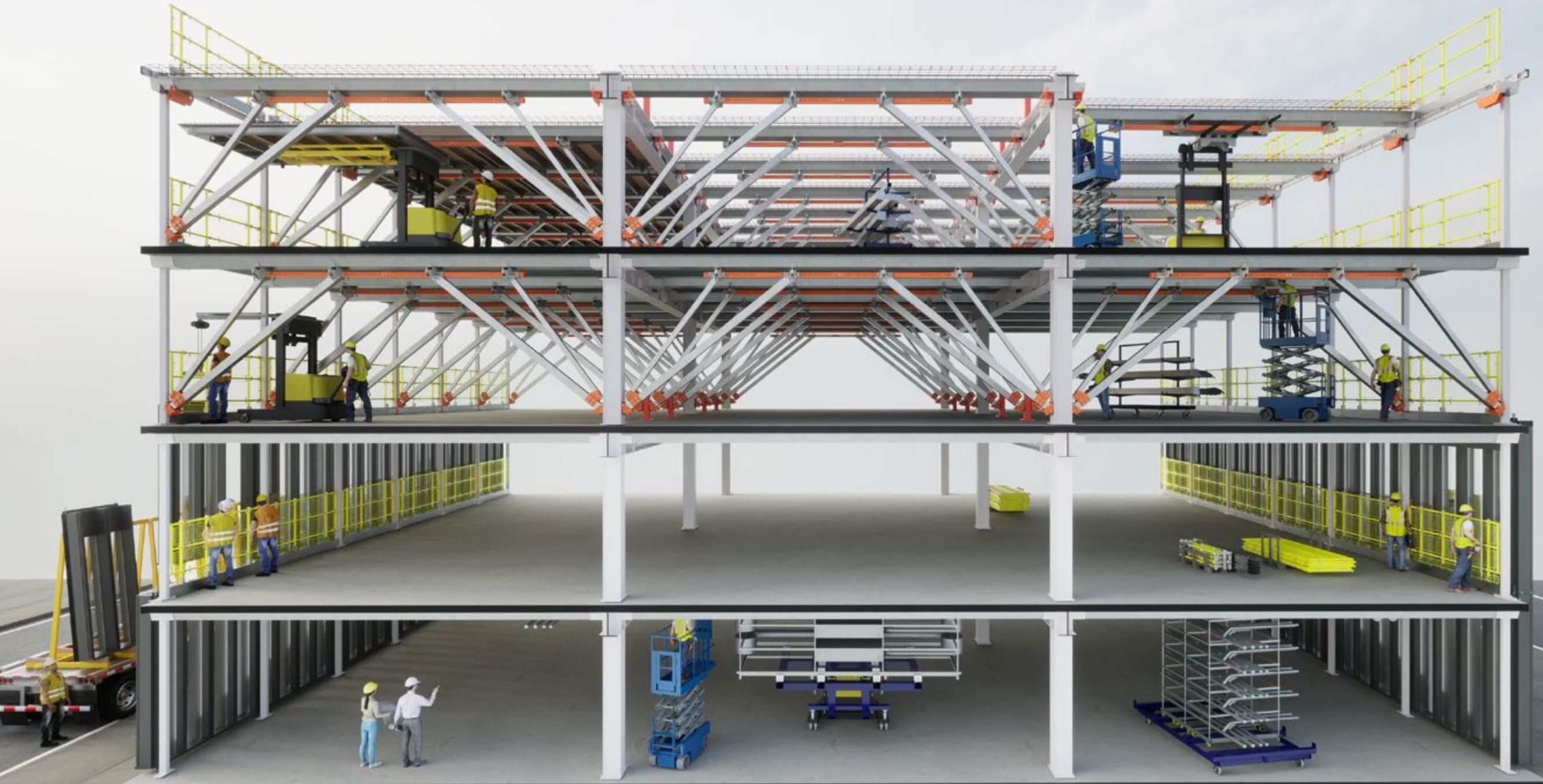
Indicative section showing key assembly processes - superstructure, façade panels and MEP cassettes.
