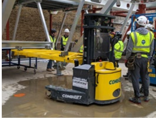
Reach stacker being used to install shutters at The Forge.
