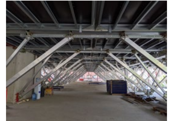
Temporary props in place at The Forge.
