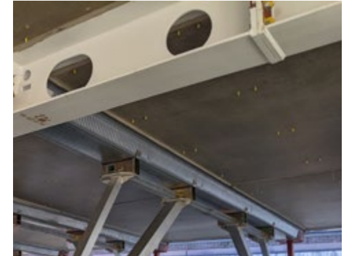
4. Completed slab soffit, with MEP fixing points visible.
