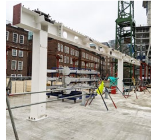
Long-span beam in place at The Forge.
