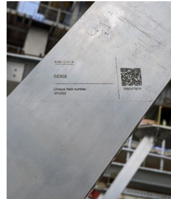
QR code etched into temporary works to facilitate tracking and reuse.
