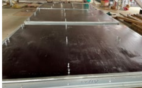
1. Shutters prior to installation - MEP fixing points are visible.
